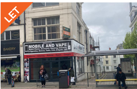
60 Western Road, Brighton
