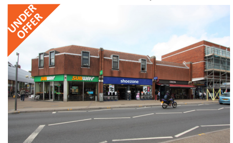
77 London Road, Portsmouth
