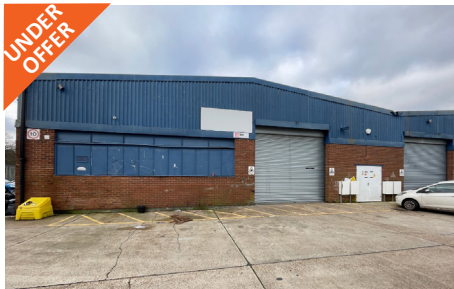
The Skill Centre, Unit 8C, Limberline Spur, Portsmouth
