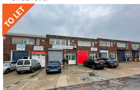
34a Aston Road, Waterlooville
