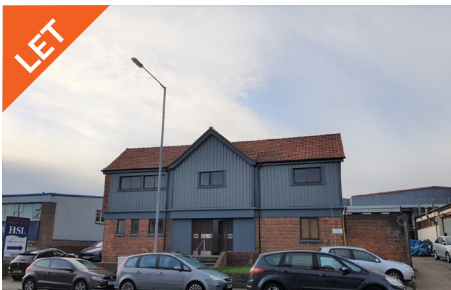
Units 1-2, Manor Industrial Estate, Newtown Road, Hove
