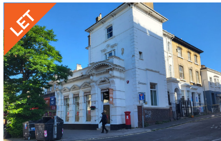
142 Western Road, Brighton
