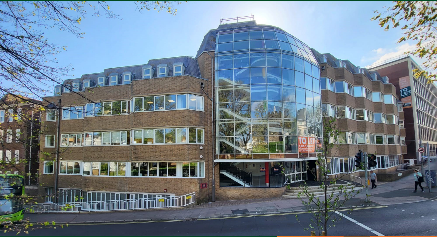
Lees House 21-23 Dyke Road, Brighton BN1 3FE
